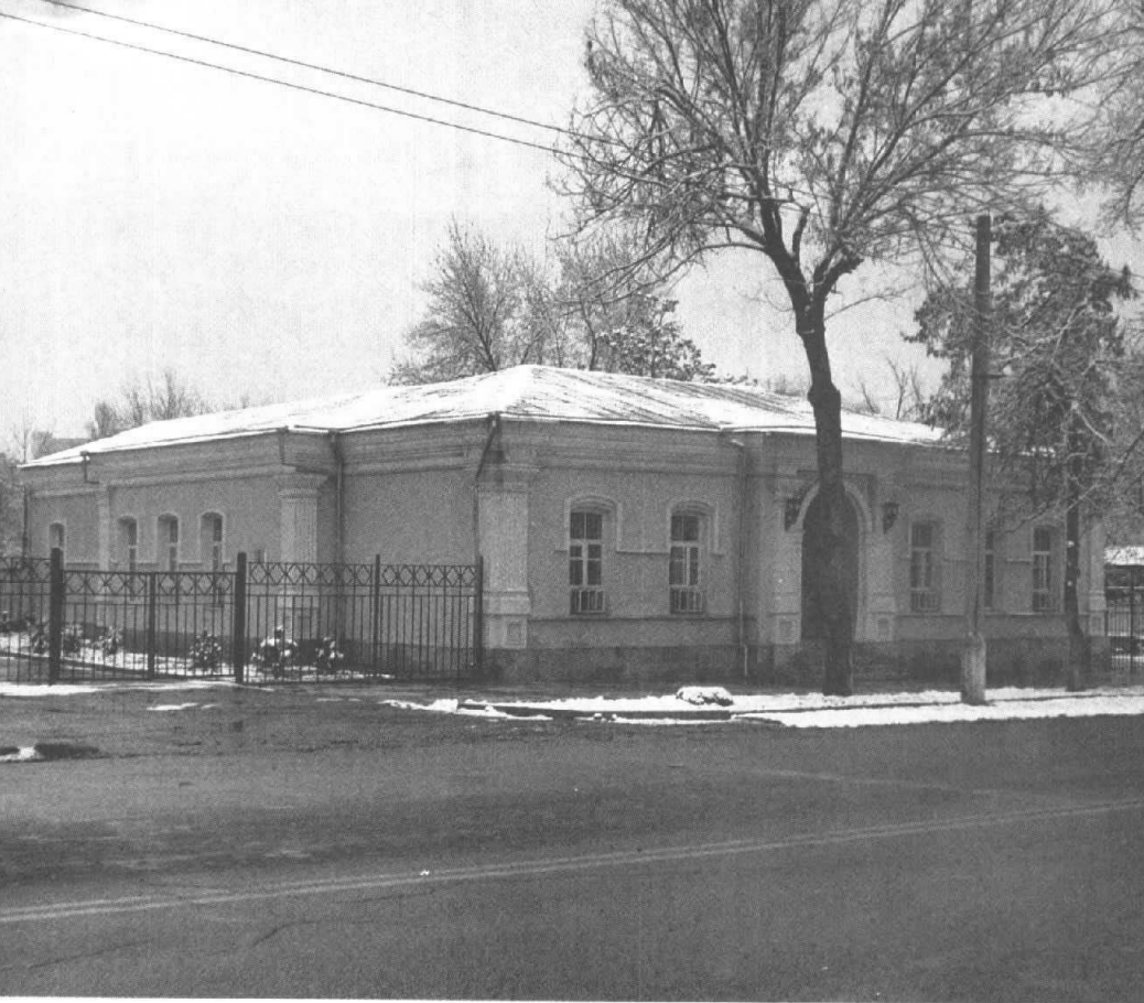
World Bank offices, Tashkent Courtesy K.S. Sangam Iyer
